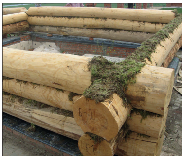
Figure 6. Traditional log-wall construction using horizontally stacked timber logs and moss insulation in a Russian izba. Source: URL: Wikimedia Commons – Log-moss-building-Reboly.jpg
