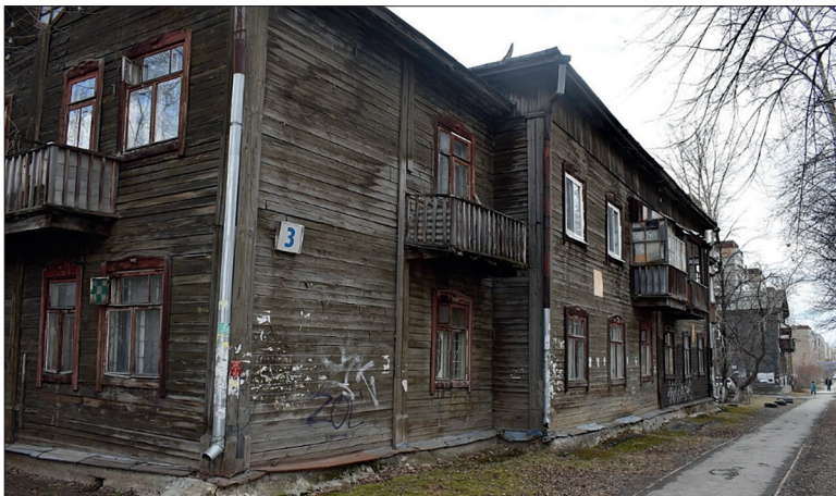
Figure 19. A two-story wooden house at 3 Uralskikh Rabochikh Street in Yekaterinburg (Ural Region), Russia, 1930's
